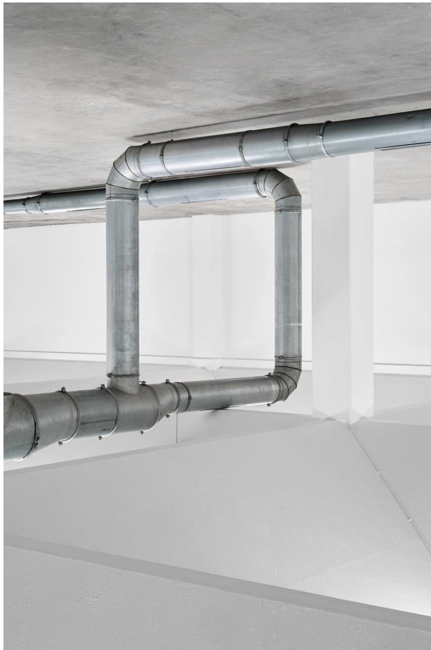
Ghislaine Leung, Violets 2 , 2018, Score : All parts of a ventilation system removed from Netwerk Aalst Bar during its 2017 refurbishment are reinstalled within the space of the exhibition and fixed from the floor, using as much of the material as possible while keeping it all interconnecting. Spare pieces that do not fit in this configuration are bracketed together in smaller formations. A welcome sign is installed. 'Fountains', 2023, installation view. Courtesy: the artist; Simian, Copenhagen, and Maxwell Graham Gallery, New York
