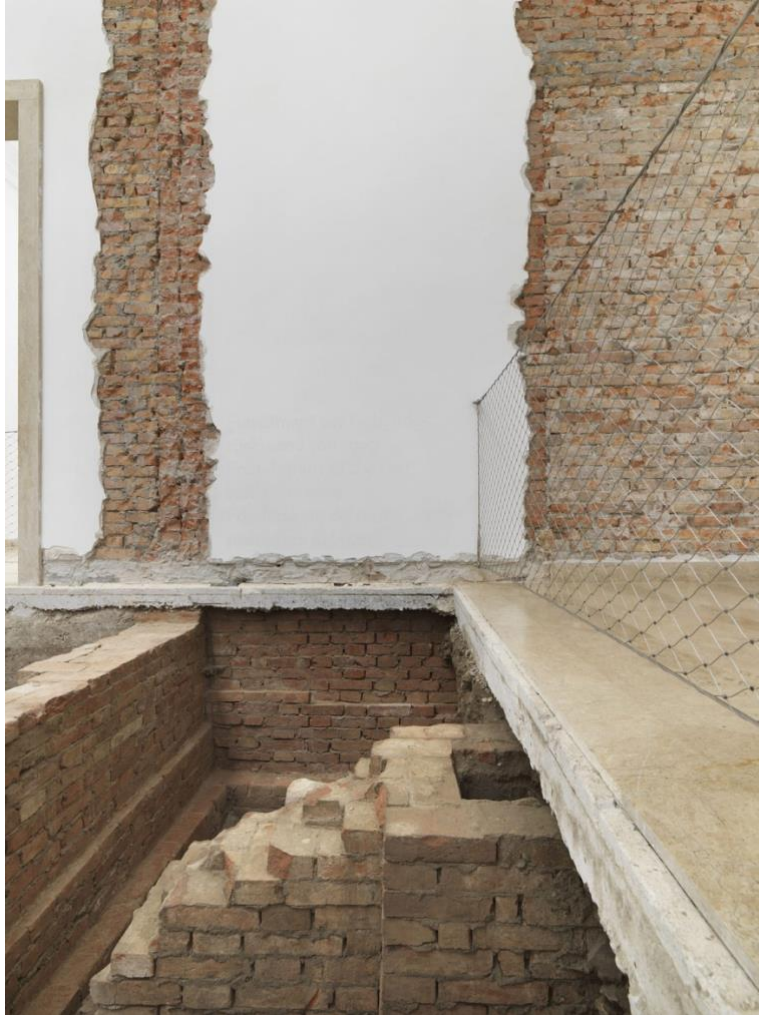
Maria Eichhorn, Relocating a Structure , 2022. German pavilion, La Biennale di Venezia. Detail: foundations of the 1909 rear facade; rear facade of the 1909 building, interior wall from 1938, demolished in 1964; wall lettering; chimney from an earlier building (undated); doorway to the right side room from 1909, bricked up in 1912. Photo by Jens Ziehe.
